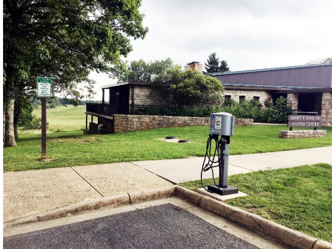
Figure 4. Charging at Shenandoah National Park. Photo by Margaret Smith, NREL 52265.
