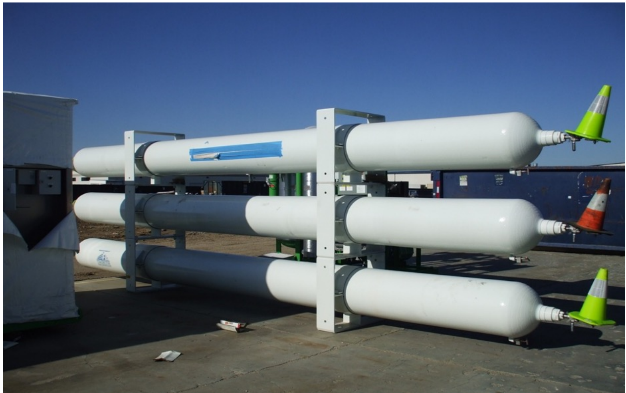
Figure 31. CNG storage vessels with three banks
