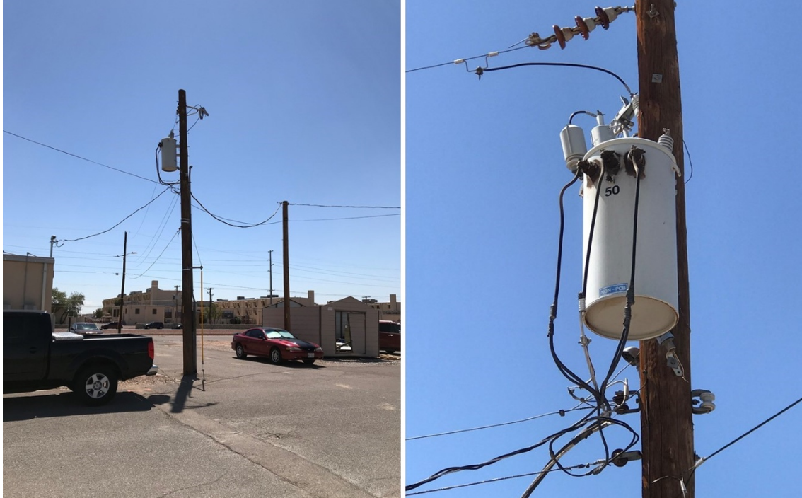
Figure 15. Single-phase 50 kVA transformer at Fort Bliss
