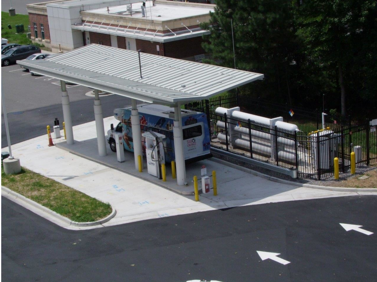
Figure 32. Example of a basic CNG fueling station Photo by Marathon Technical Services, NREL
