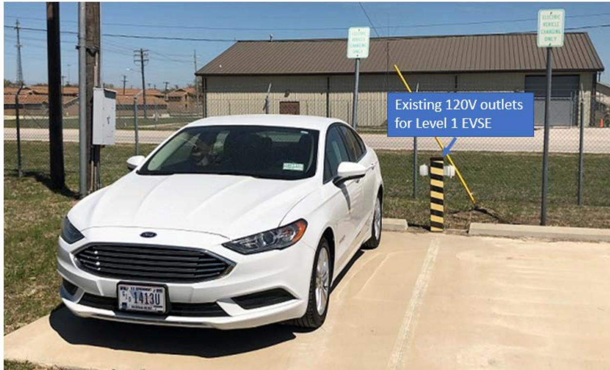
Figure 25. Dedicated parking space with existing Level 1 at North Fort Hood TMP
