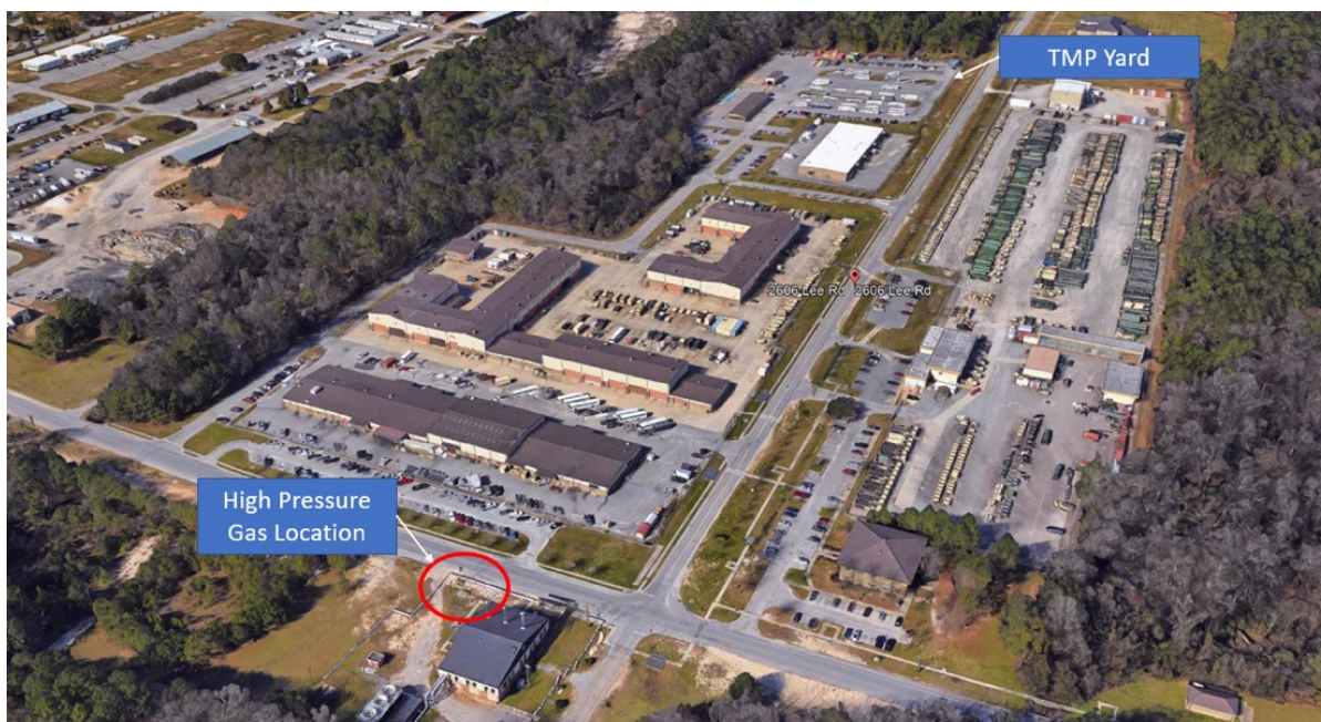
Figure 26. TMP yard and high-pressure gas location at Fort Jackson
