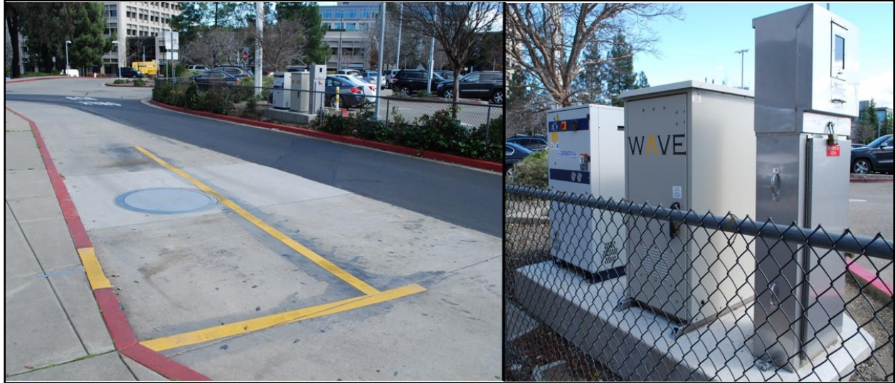
Figure 2-4. WAVE inductive charging pad (left) and charging equipment (right)
